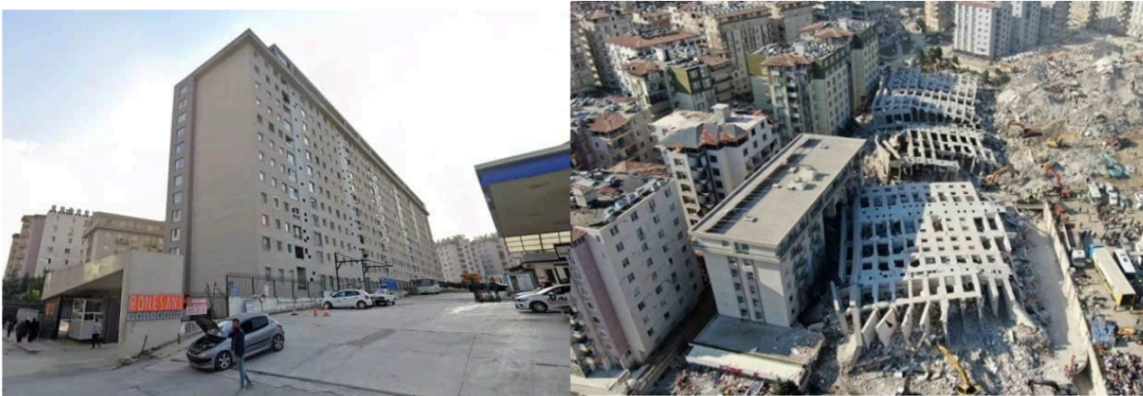
Figure 1. Rönesans Rezidans Before and After the Earthquake Collapse.
