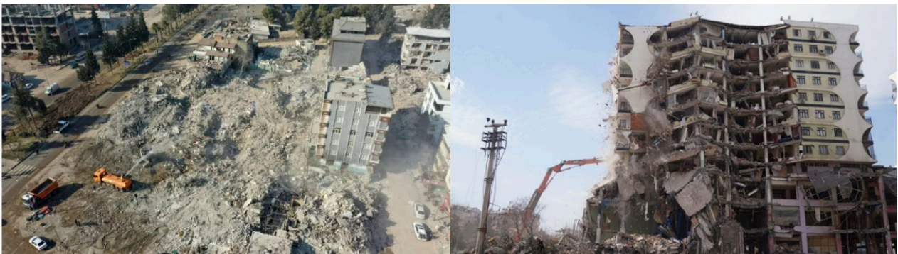
Figure 3. Isias Hotel Before and After the Earthquake Collapse.
