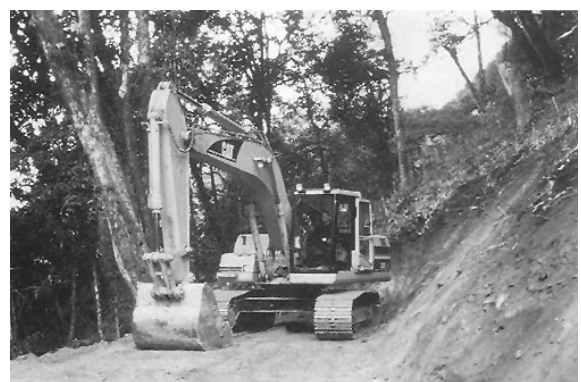
Figure 1. Road smoothing by means of the bulldozer's blade (Left) and excavator's bucket (Right).
