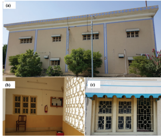
Figure 1. (a) Windows of office-2 (b) Windows of office-1 and (c) fixed over hang shade
