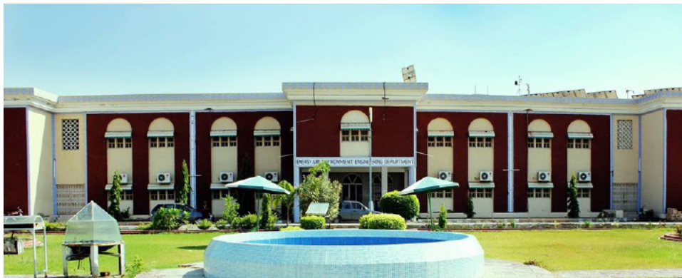
Figure 1. A view of Energy and Environment Department
